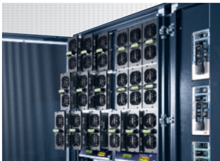
Archimod UPS with “hot swap” system
